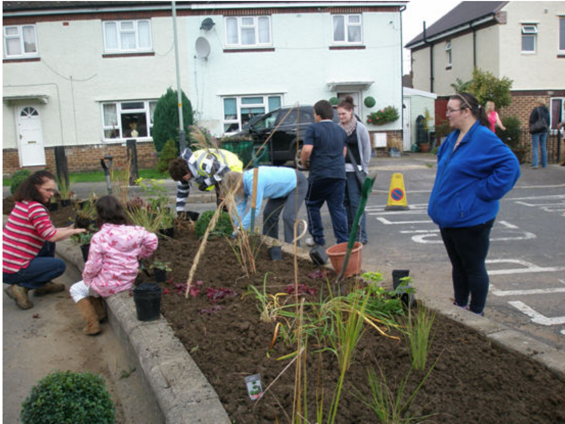
Humber Road streetscape improvement, Oakley
