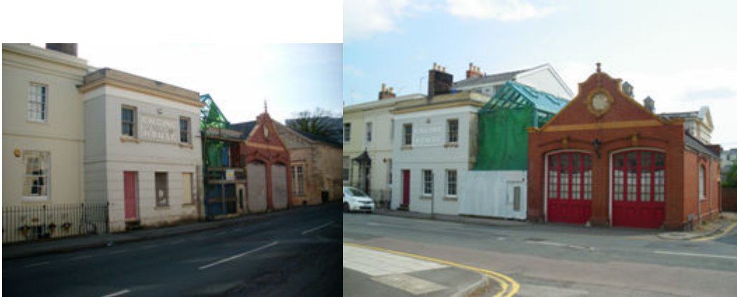
Results of enforcement action, Old Fire Station, Jessop Avenue
