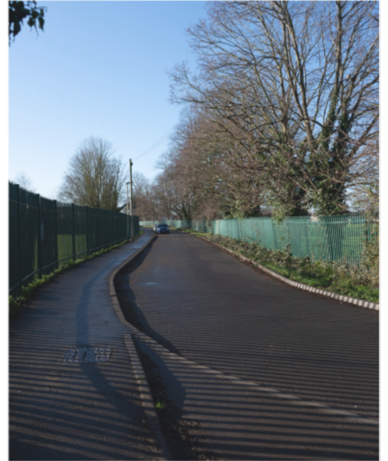
Photo 06 - Top of Gardners Lane looking South
