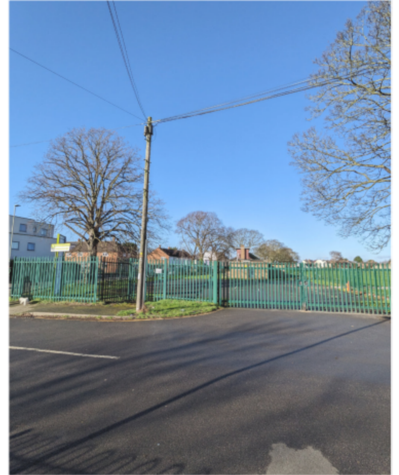
Photo 09 – Existing car park entrance, Gardners Ln
