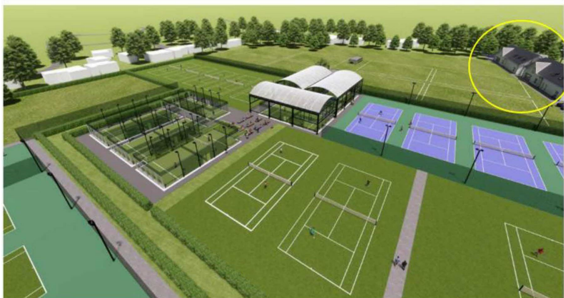
East Glos Club Padel Courts
