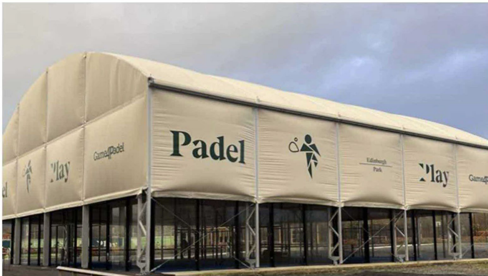
Installation in Edinburgh
