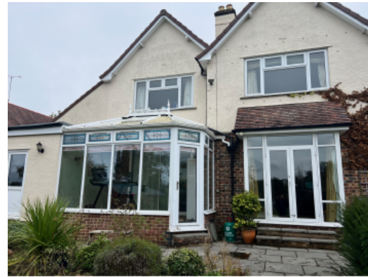
Rear of no.187
