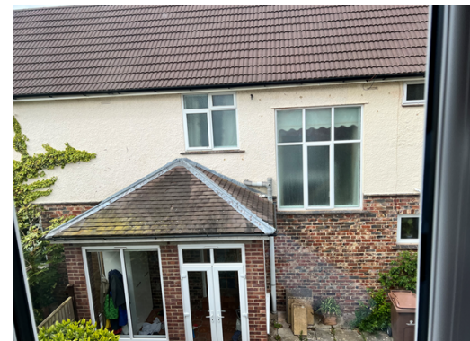
View from first floor side window of no.189 looking towards no.187
