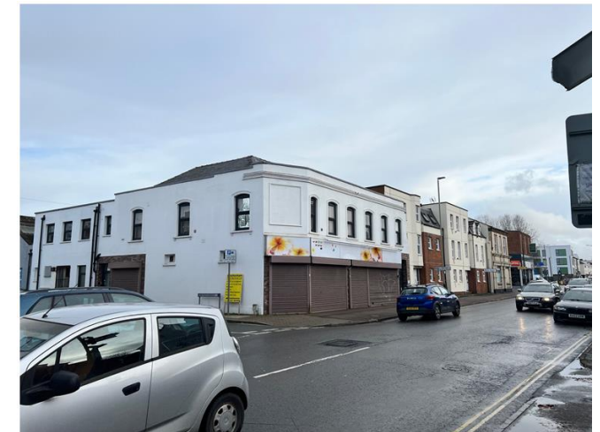
449 - 451 High Street (diagonally opposite the site to northeast)
