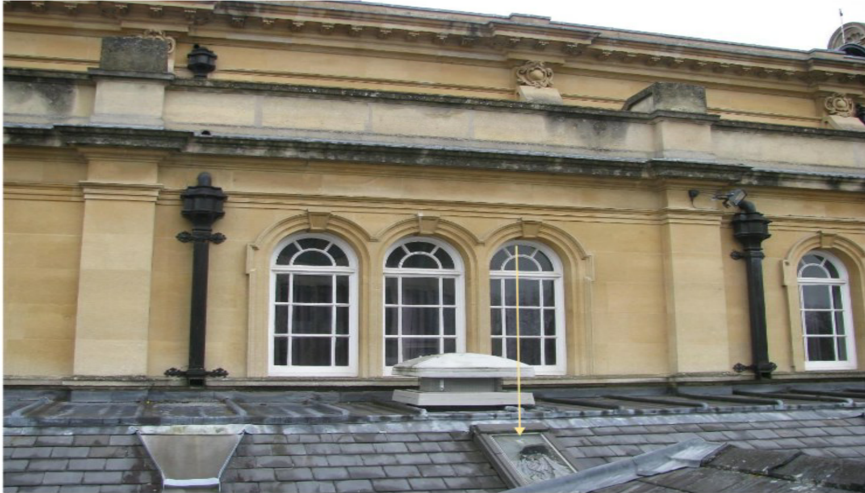
Figure 1. View of First floor roof with broken skylight (1 of 5 skylights). All the skylights are located along the pitched slate roof on this west elevation.
