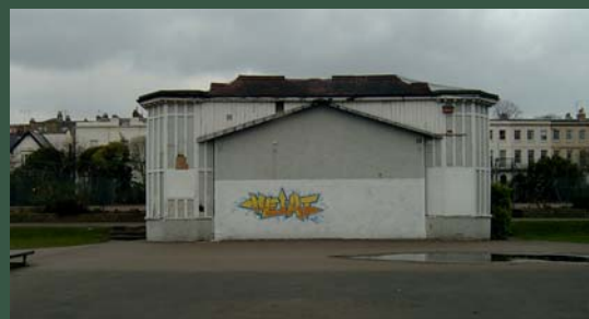
1999 : The brick built Gymnasium was removed 1999/2006 : The Proscenium fell into disrepair
