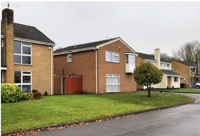
7) Street view of No.'s 15 & 17 (front apex/gable) and then No.'s 19 & 21 having forward extensions with render.
