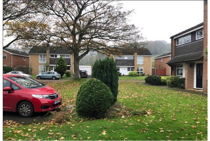
6) 16 Hartley Close looking at No.'s 11 & 15 with front porch to the right
