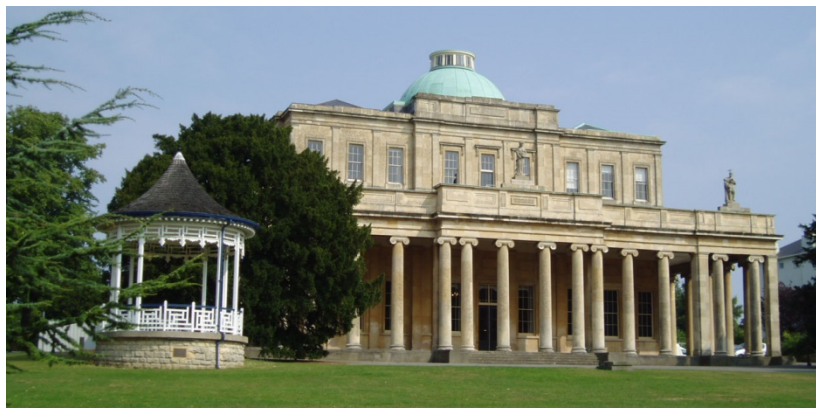
Pittville Pump Room
