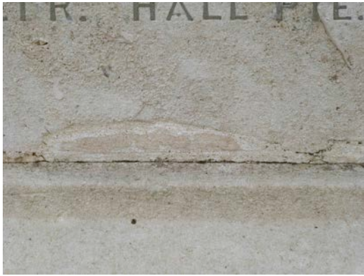
Fig 20: repair at base of inscription panel
