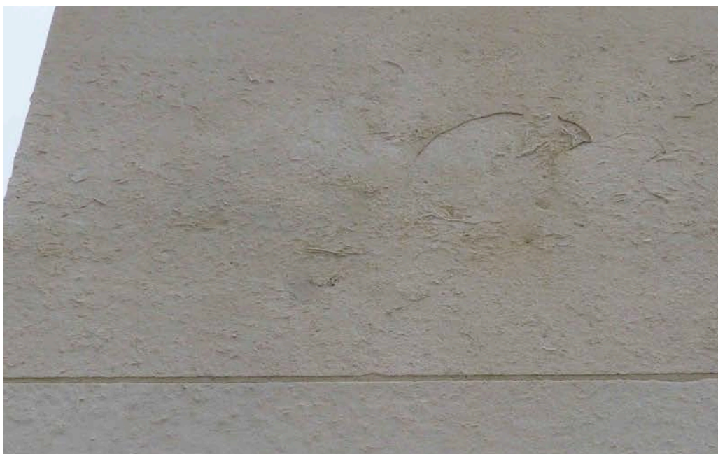
Fig 12: detail of obelisk stone showing how shells (which do not erode) stand proud of adjacent eroded stonework
