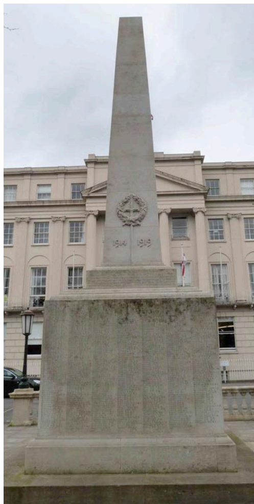
Fig 22: overall view of east elevation
