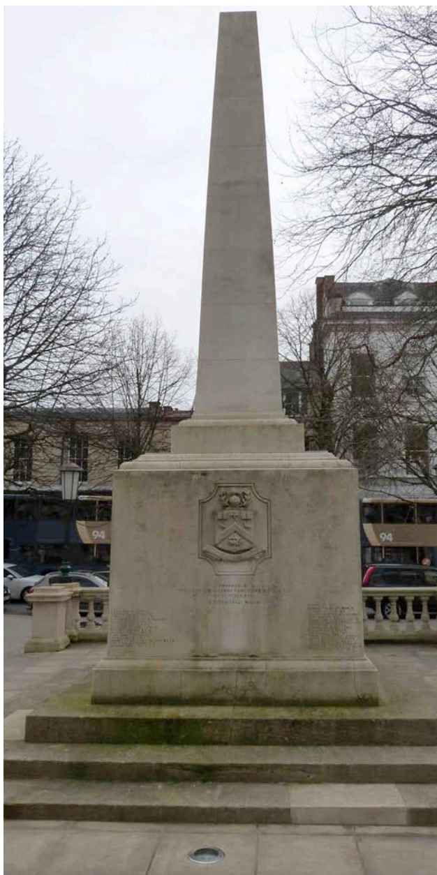
Fig 32: overall view of west elevation
