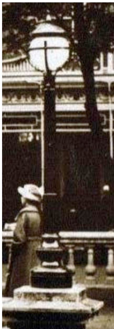
Fig 56: detail of original lantern
