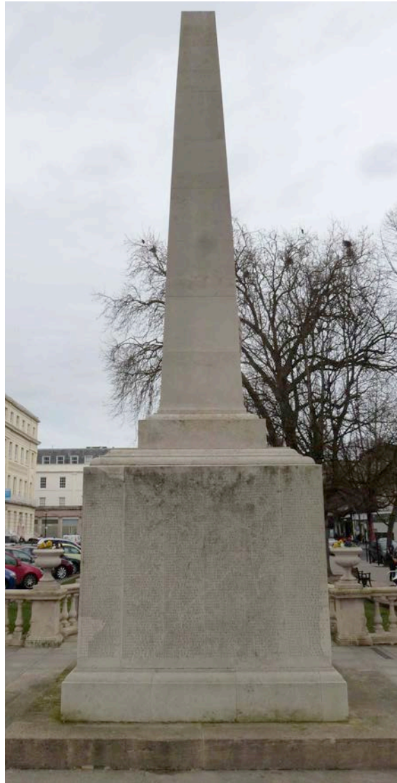
Fig 18: general view of south elevation
