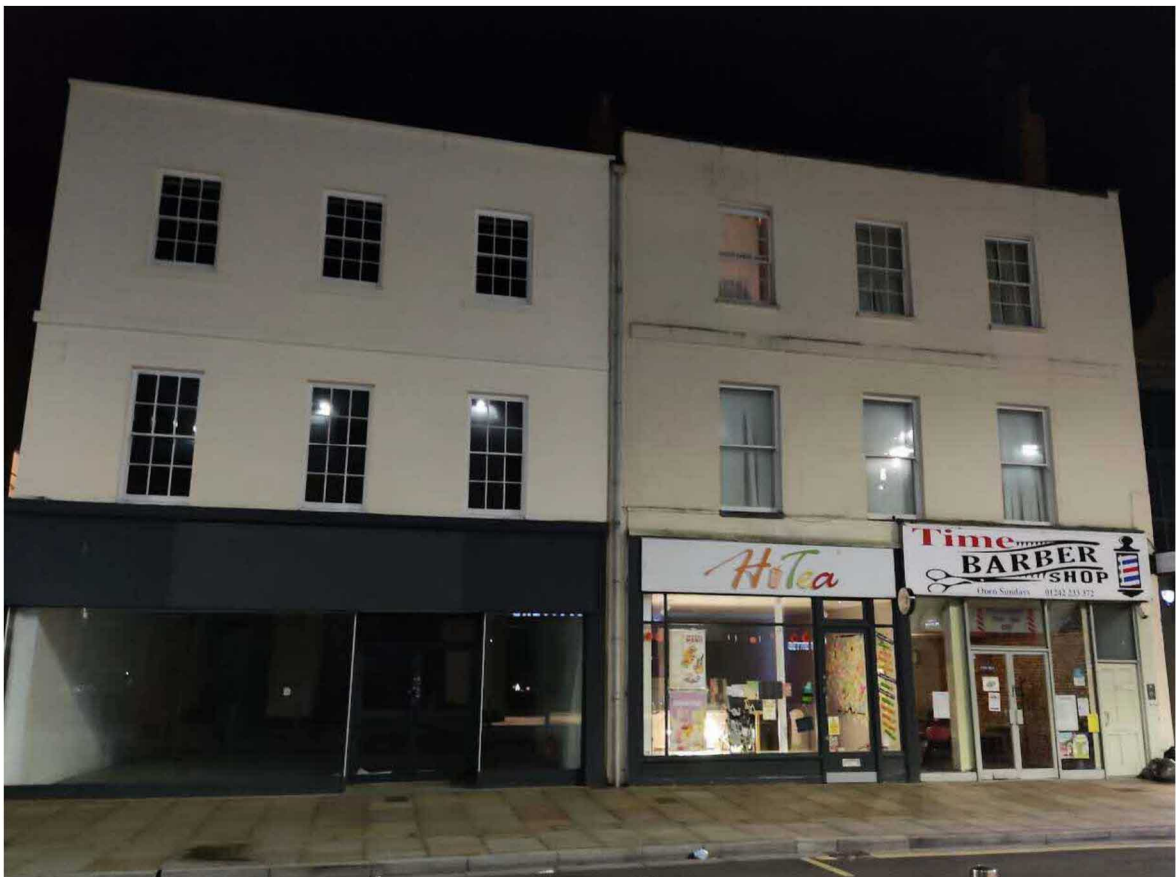
Figure 7: Residential use above 220 and 222 High Street are structurally connected to the appeal site presenting a higher risk of structureborne sound transmission from the proposed change of use.
