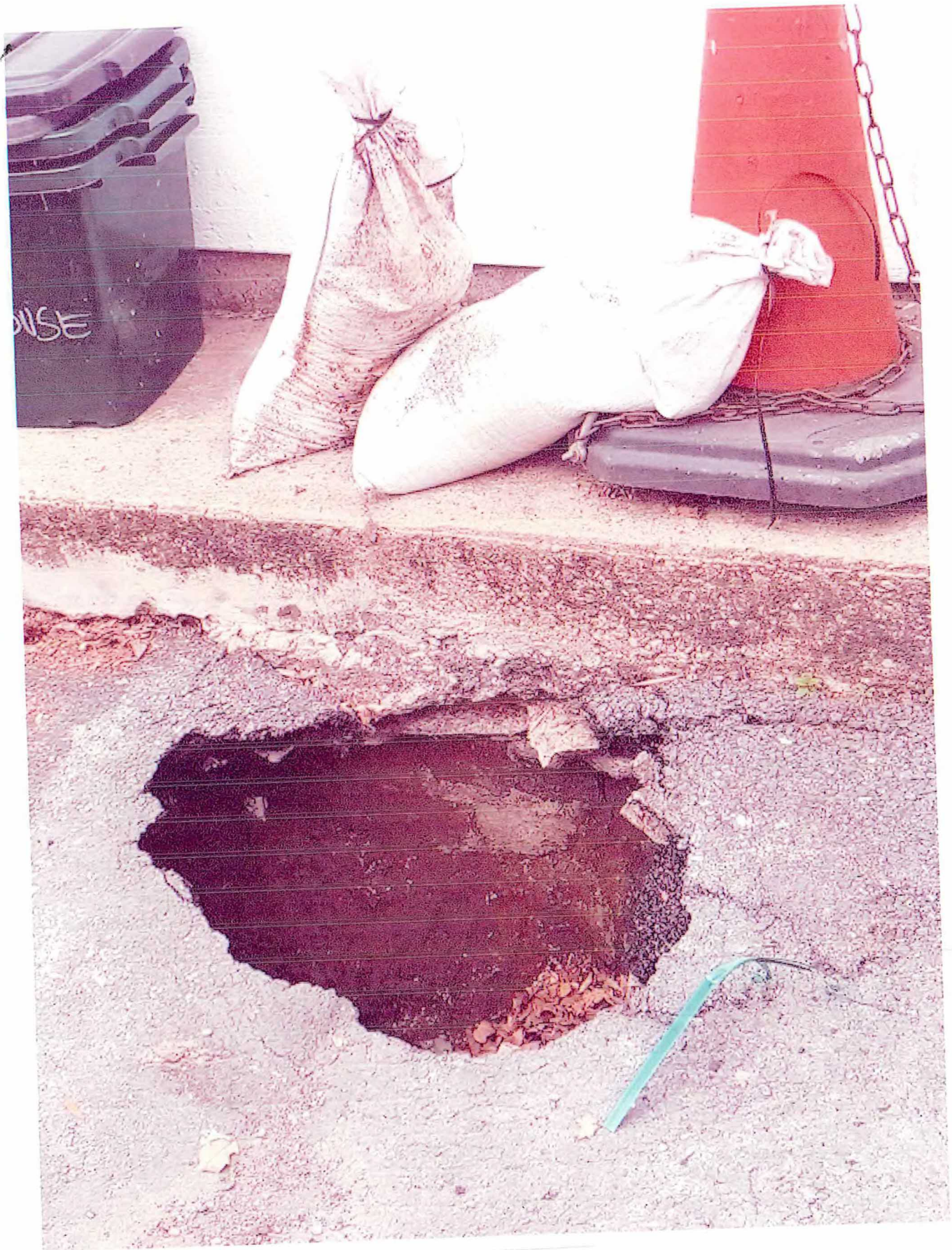
COLLAPSE OF SUBSTRUCTURE OUTSIDE THE OLD COACH HOUSE WELINGTON LANE
