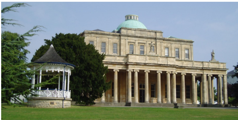
Pittville Pump Room
