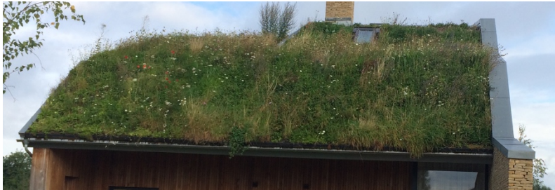
Green roof on a low carbon house in southern Gloucestershire
