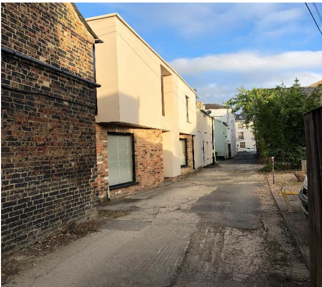
CHURCH WINDOWS IN POOR CONDITION
