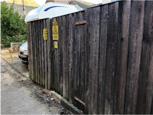
ROAD IN POOR CONDITION
