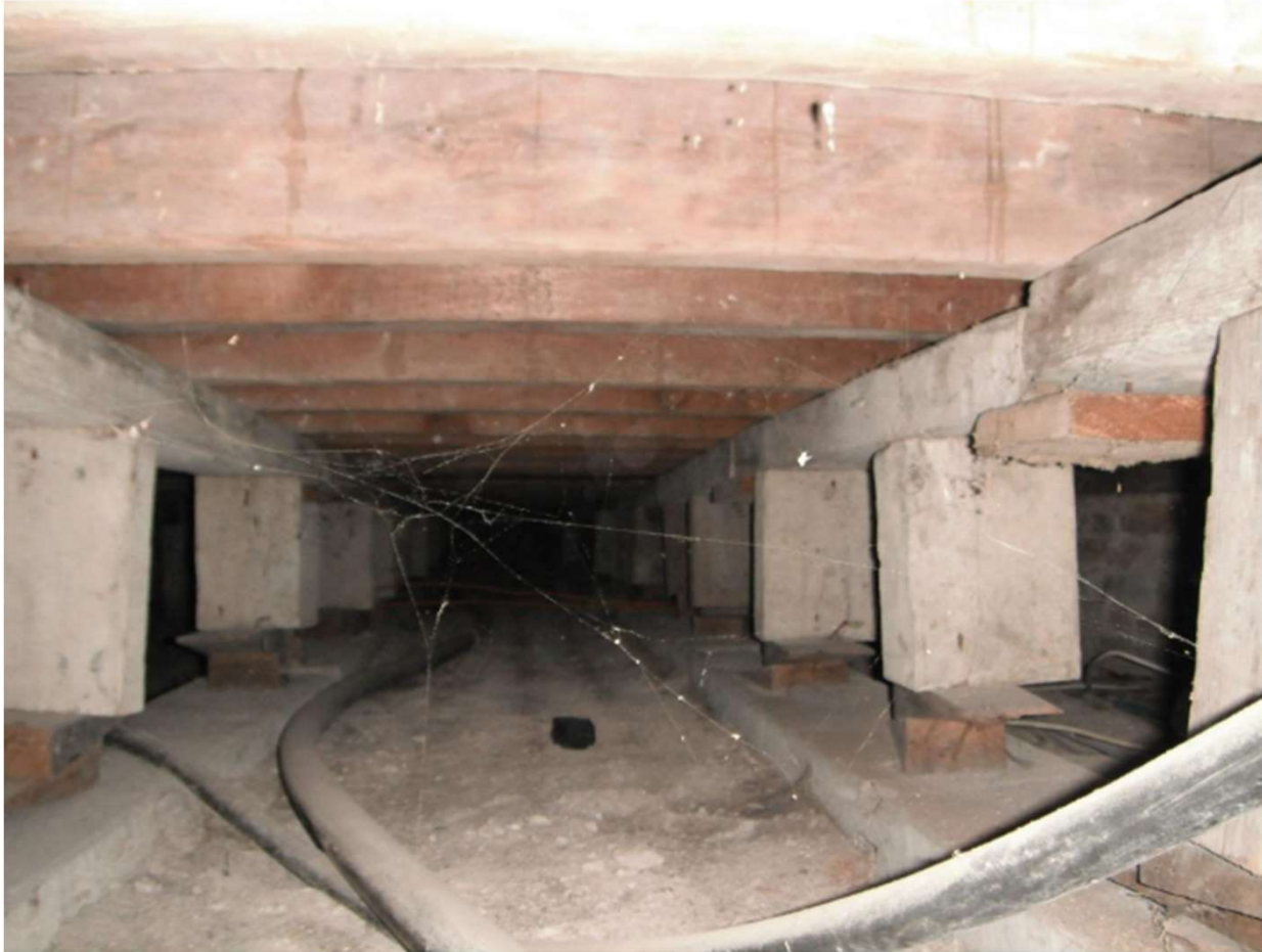
Figure 6. Existing floor void: Two lines of floor support props with folding wedges under, onto a timber plate in turn onto a rough concrete base. The floor joists are on top of a timber plate which is fixed to the props. The boarded floor is over the top of the floor joists.
