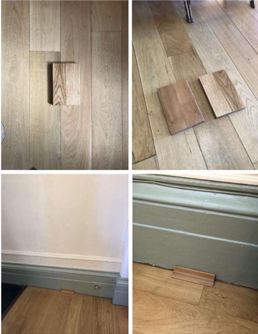
Figure 7. Top left photo: Junkers oak sample against existing flooring. Top right photo: Junkers oak sample (right) beech sample (left). The oak is proposed for the new floor. Bottom left and right photo: Proposed skirting to cover expansion gap required on the new flooring.
