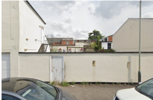
A) Google Street View of rear of building from Oakland Street
