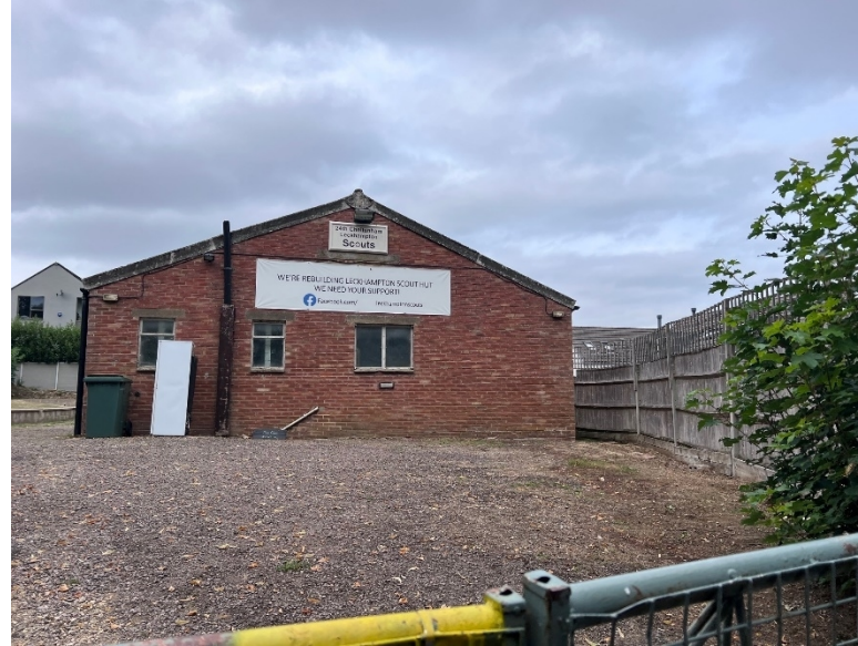
Existing building (east elevation)
