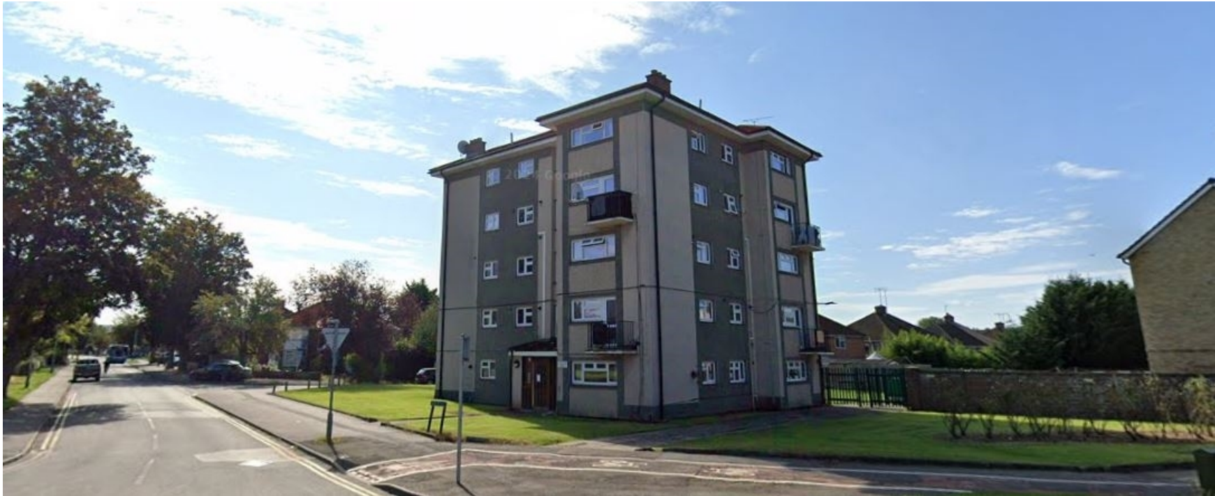
Existing Site Photo
