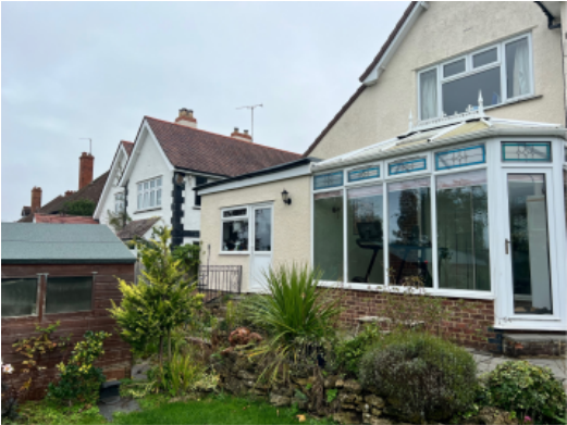
View from rear garden of no.187 looking towards no.185
