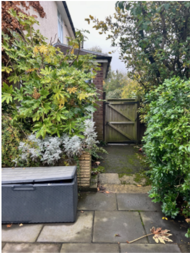
View of the side of no.187 from the rear
