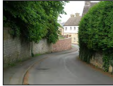
Figure 12 Traditional boundary treatments evident in Mill Street
