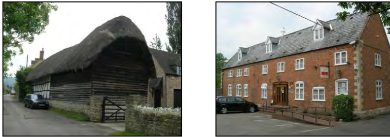
Figure 22 Historic barn on Lake Street and former stables of Prestbury House
