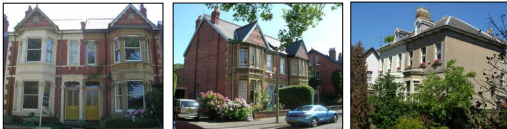
Figure 19 Unifying architectural detailing on houses
