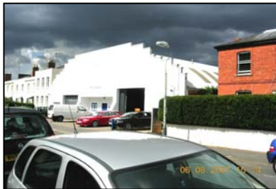
Figure 22 Depot in Carlton Street
