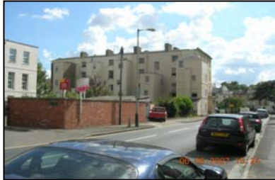
Figure 13 High brick wall at the rear of Berkley Place
