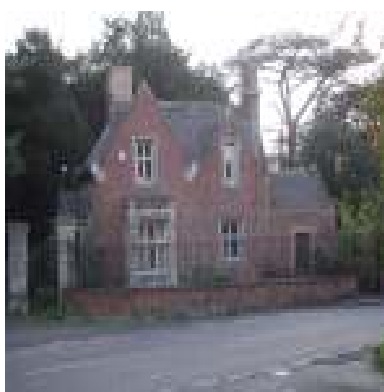
Fig. 11 Swindon Hall Lodge
