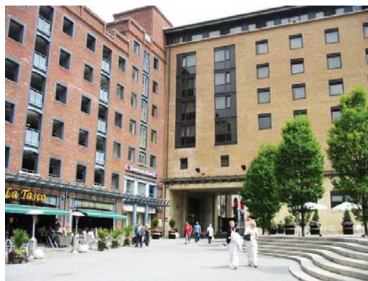
Figure 6: Example of multi-storey car park (left) overlooking public space
