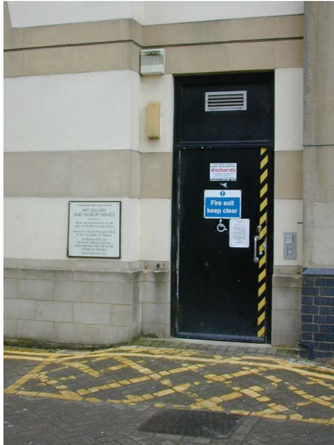
Ramped approach to the rear of the building. Chester Walk.
